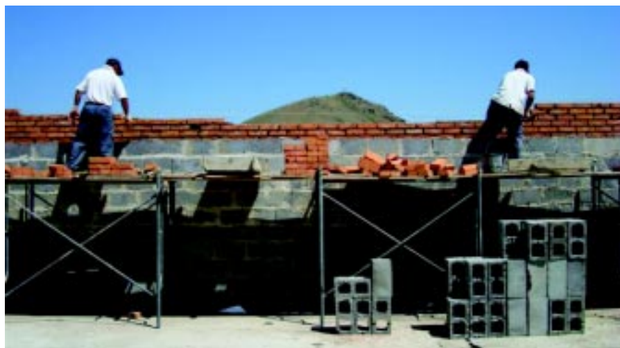
Arts & Music Theatre under construction, Blue Skies Ger Village, Mongolia
