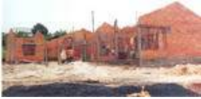
PHOTO: The Construction of Gung Re School
